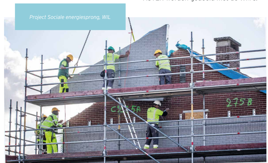
*Ressorts (fr), Stichting global energiesprong alliance (nl) Buro de haan informatie technologie bv (nl), Pouget consultants (fr), Nobatek (fr) Ene-project (de), Edera (it), Atnaujinkime miesta (it), Roofuz (de), Renowave (at), Saxion university (nl), Delta ecopolis (it), Buildup (be), Institut fur nachhaltige technologien (at), ASTER (be), Wonen in limburg (be), Alliade habitat (fr)
